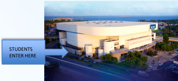
Pensacola Bay Center front (west) entrances
