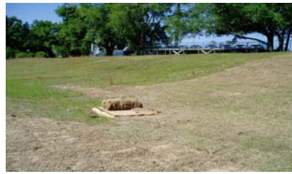
Drainage pipe area with new inlet
