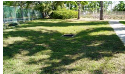
New Drain Inlet
