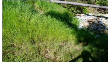
Outlet with Rip Rap
